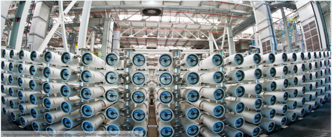
https://genesiswatertech.com/wp-content/uploads/2019/08/RO-waste-water-recycling-1.jpg Ters Osmoz Sistemi
